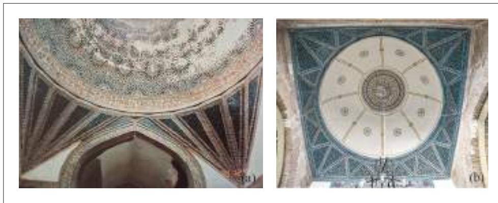
Figure 6. (a) The transition element with fan pendentive in the closed courtyard of Karatay Madrasa in Konya (Boran, 2001; figure 539) and (b) the belt of Turkish triangles of Alaaddin Mosque in Konya (Bilici, 2016a; 23).
