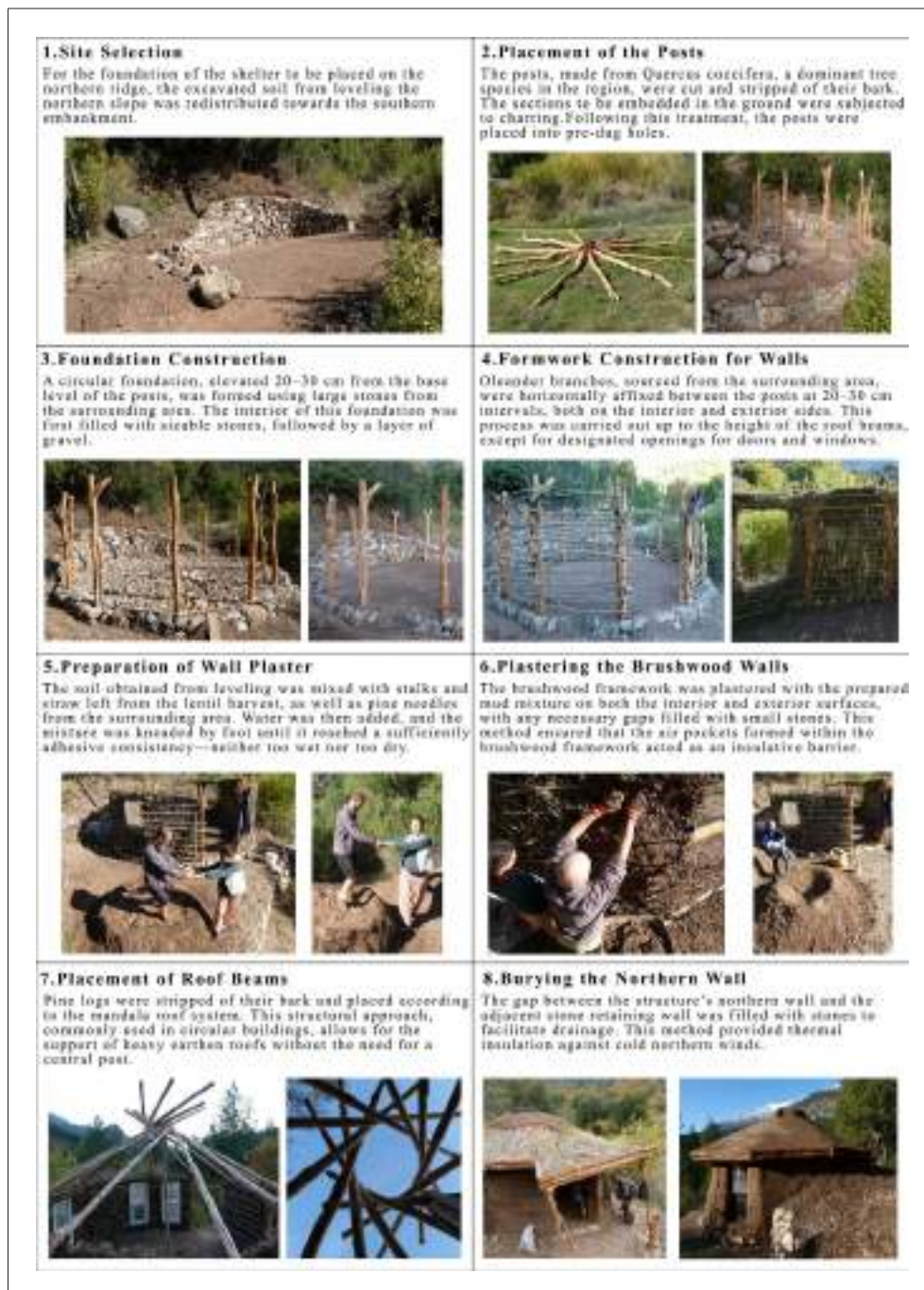
Figure 4. Sequential construction phases of the earthbag 'Yuva' prototype (Erkutlu, 2012).
