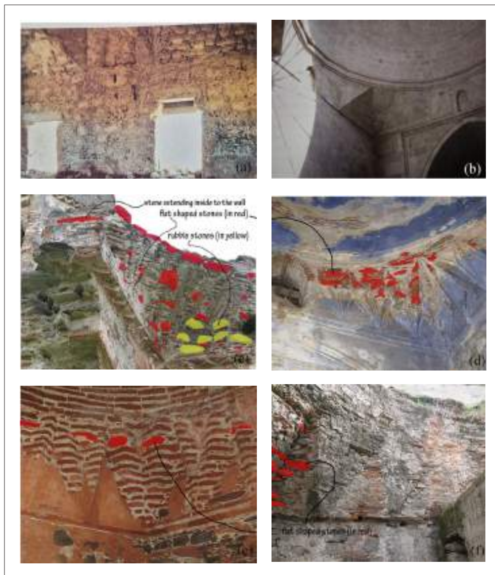
Figure 15. Stone usage; (a) Yanköy İçkale Masjid in Antalya (Boran, 2001; foto 224), (b) Vacidiye Madrasa in Kütahya (Kolay, 2017; 59), brick and stone hybrid usage; (c) Molla Arap Mosque, (d) Yalınayak Masjid, (e) Tahtakale Bath and (f) Karagazi Bath in Tire (Author, 2007).
